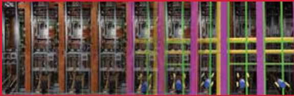
Piping within the walls of the Omaha Public Library, overlaid with a virtual model built with Blender.
